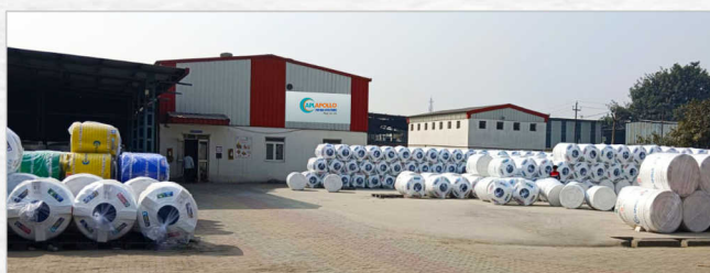
Manufacturing Plant - Sikandrabad (U.P.)
